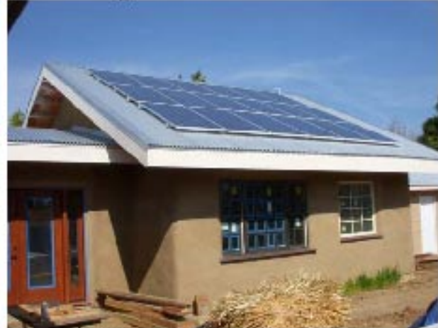
Owner-builder project in Vista
