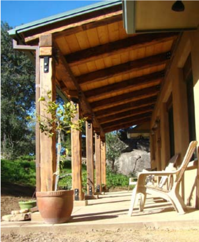
The south-facing porch with vintage timbers.
