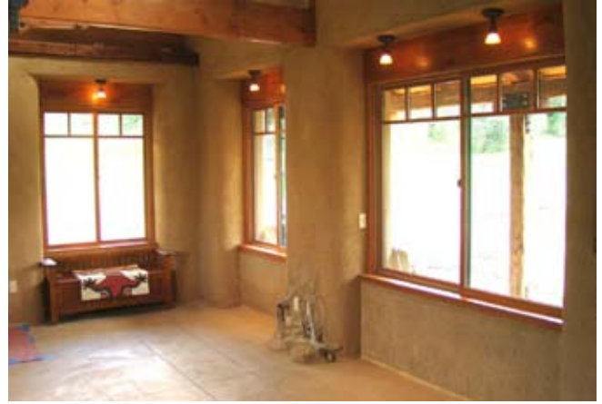
Heavy wood lintels and gracefully plaster radii frame the windows.
