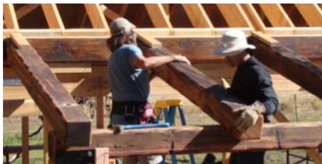
Builder & CASBA member Paul Turner positioning a vintage timber.
