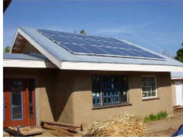
Owner-builder project in Vista
