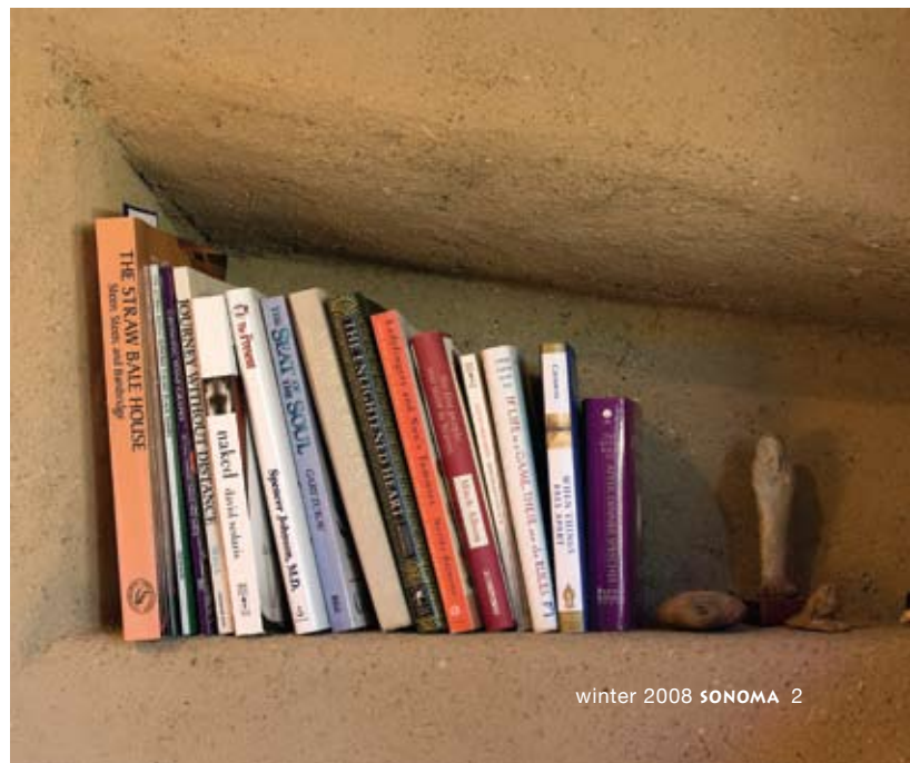
Straw-bale walls allow numerous niches, including the traditional "truth window" that exposes the home's building material.
