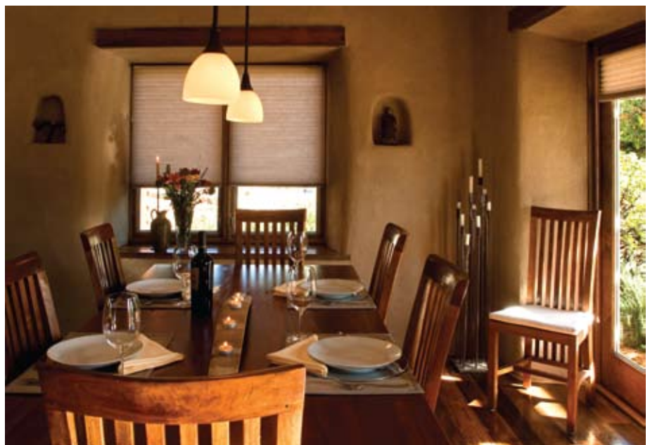
Doorways and window sills reveal the 35-inch-wide walls that provide superb insulation and interior silence.
