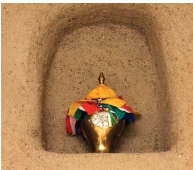
Straw-bale walls allow numerous niches, including the traditional "truth window" that exposes the home's building material.
